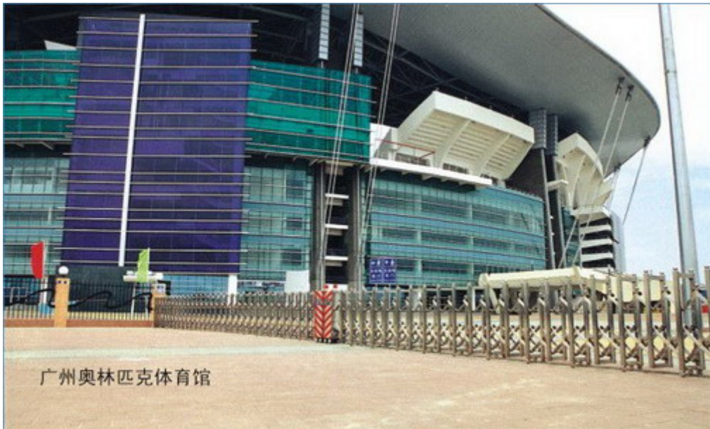
Pic 5. Guangzhou Olympic Stadium (Folding Gates)
