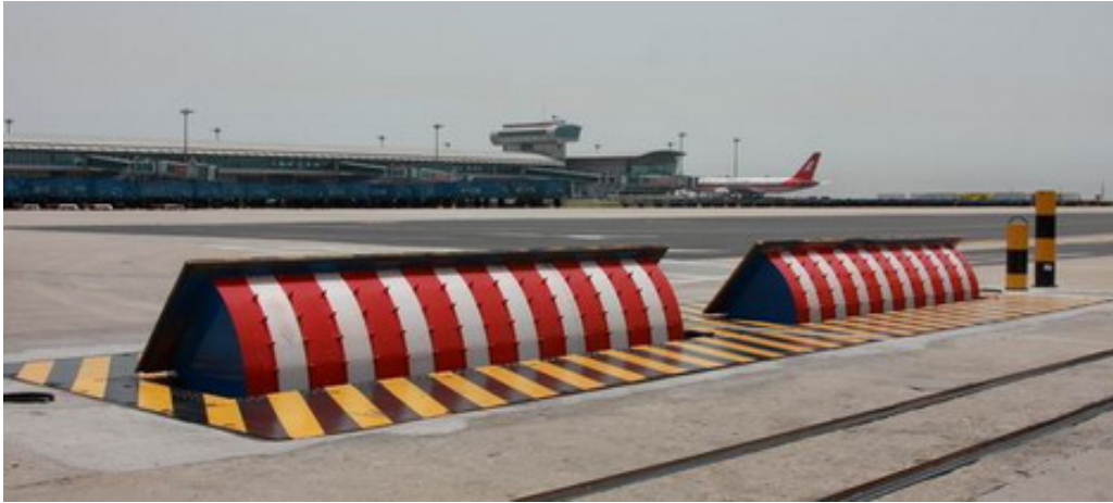
Pic 4. Shenzhen International Airport (Road Blockers)
